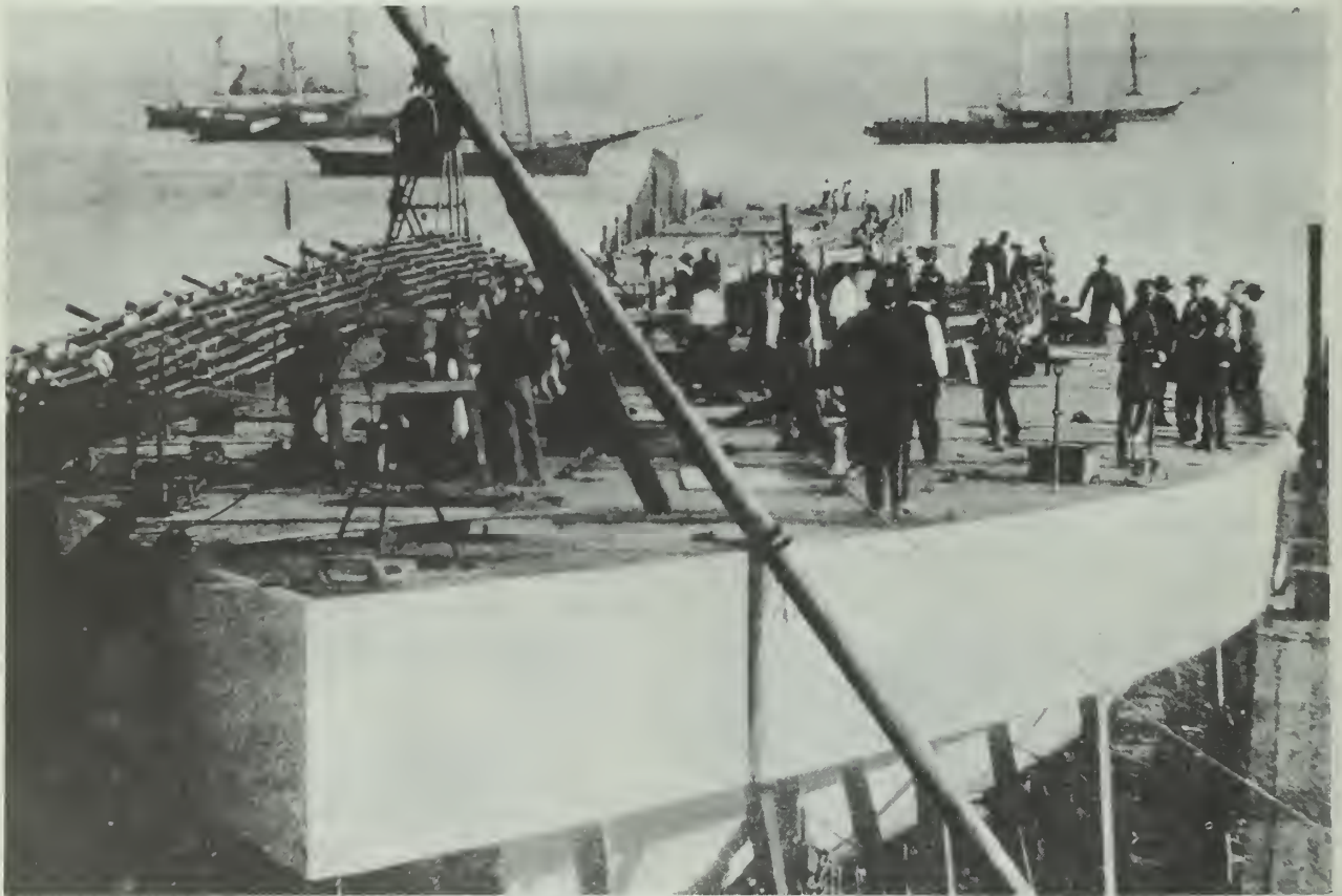
U.S. Monitor Camanche under construction in San Francisco during 1864—This photograph appears to have been taken shortly before the one on page 762 as the ships in the background are the same.
